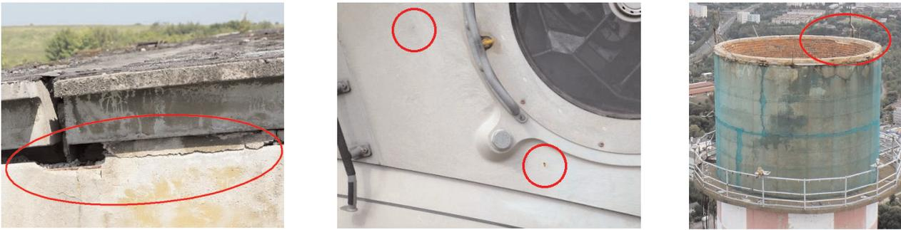
**Figure 5.** Examples for possible image quality: cracks in a wall roof joint (left,  $h = 15$  m,  $L < 5$  m), rusty spots on wind turbine machine house (centre,  $h = 100$  m,  $L \approx 10$  m), damages on inner brick lining of a chimney (right,  $h = 225$  m,  $L \approx 25$  m)
