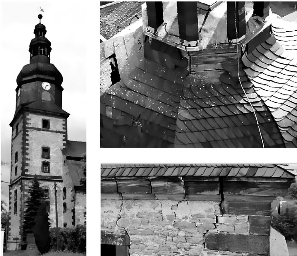
**Figure 4.** Masonry church 44 m (left), detected slate roofing damages (top right, elevation  $h = 40$  m, object distance  $L \approx 10$  m), detected critical cracks at masonry corner roof joint (bottom right,  $h = 25$  m,  $L \approx 5$  m)
